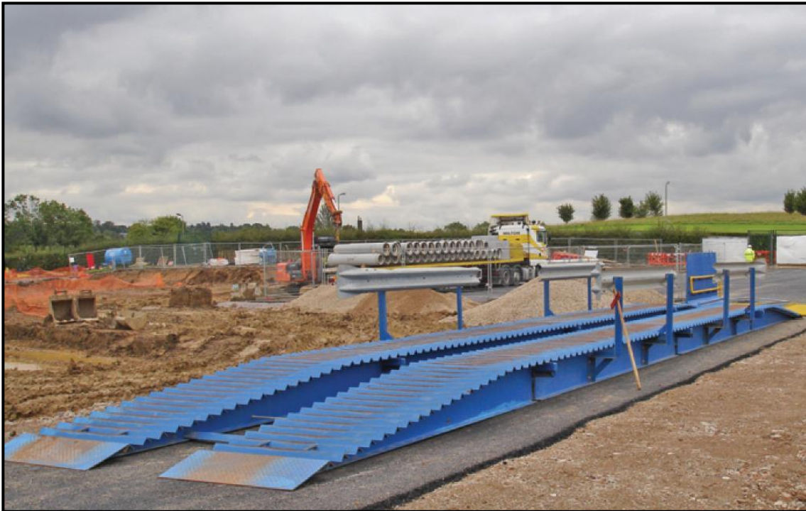
Figure 3-1 Typical wheel wash using the dry ramp system
